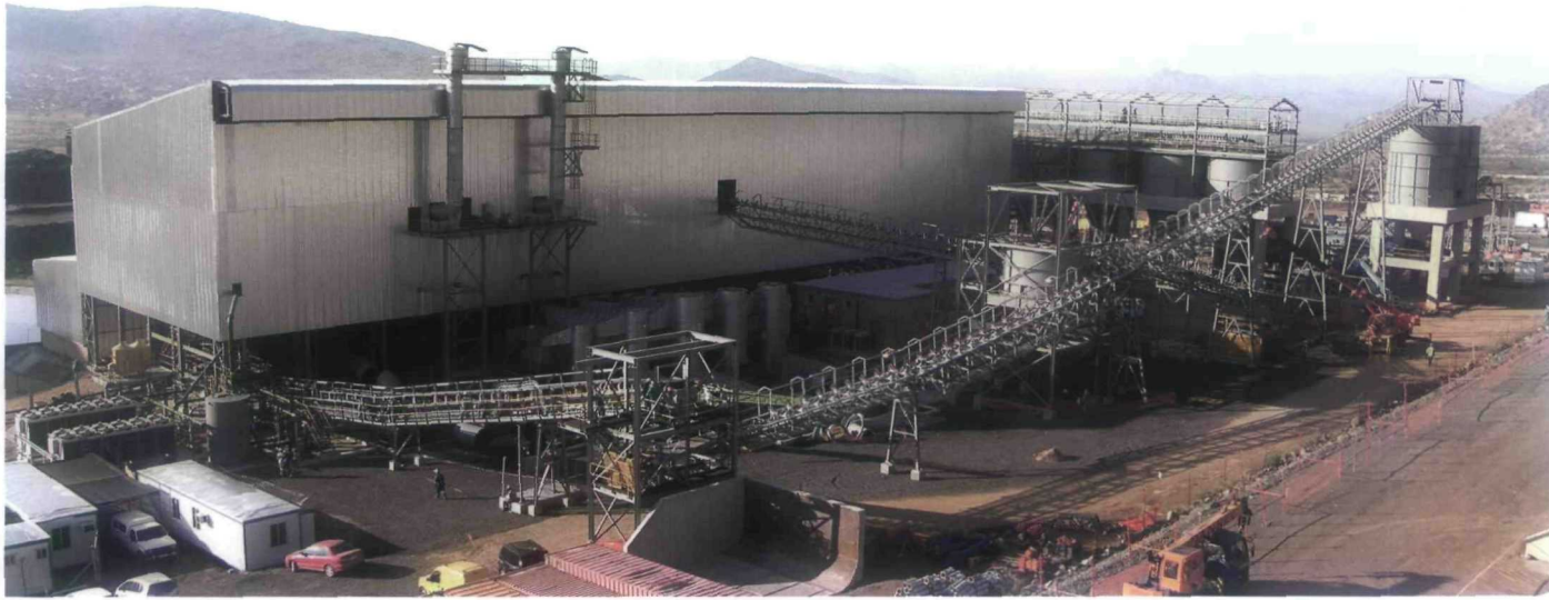
The Burgersfort site photographed in May showing the main sinter building and pellet handling section (photo: Metix).
