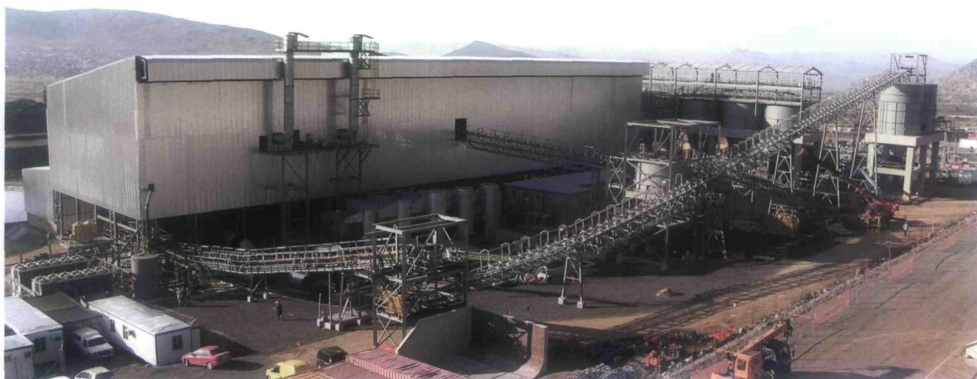
The Burgersfort site photographed in May showing the main sinter building and pellet handling section (photo: Metix).
