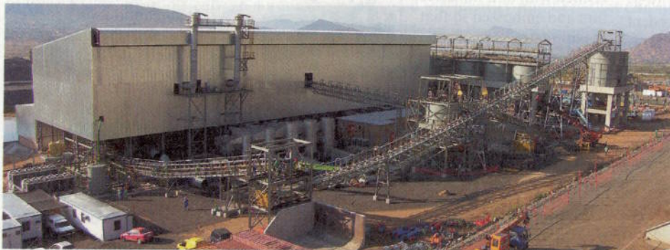
NEARING COMPLETION ASA Metals' pelletising and sinter plant
